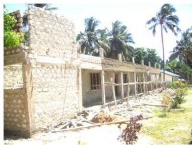
New 4 Classroom Building at New Life Academy
